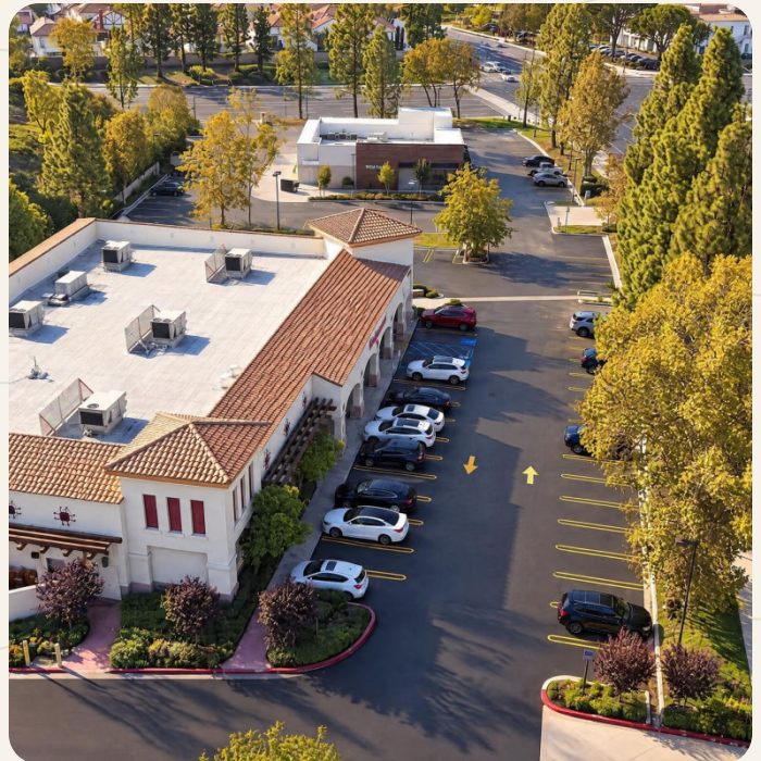
The shop building from the parking field, and Walgreens with the greenbelt slope behind.
