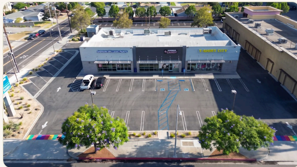
The Suite C storefront and the three tenant building. Photos digitally retouched.
